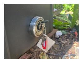
5. Turn the allen key, this should set the gates in to manual to allow them to be pushed open.
